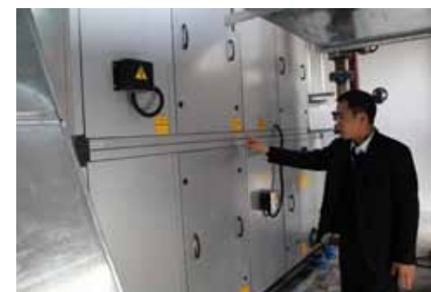
佛山分行“绿色建筑”：热回收循环风机 “Green building” of Foshan Branch: Heat recovery circulating fan
